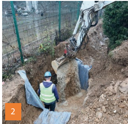
2 Material filling for the chamber foundation.
