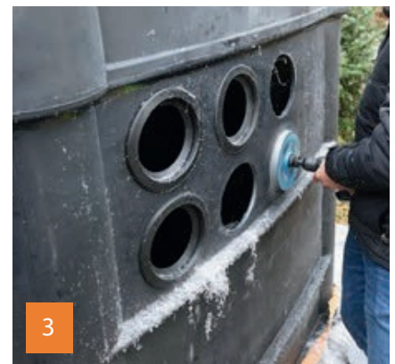
3 Installation of the connections to the chamber.
