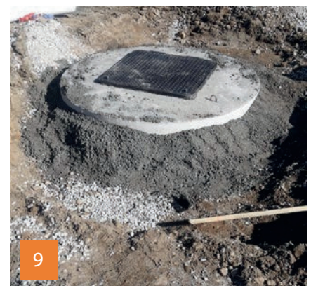
9 RC ring successfully installed.
