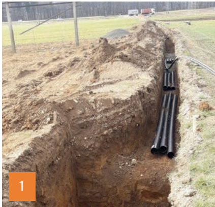
1 Preparation of the construction pit.
